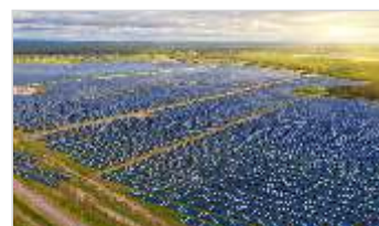
2012MWp Jindal Renewables Bikaner, Rajasthan (Under Commissioning)
