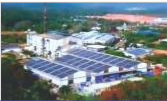
1700KWp Pirmal Glass Ltd. Gujarat
