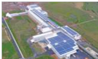
2000KWp Mondelez India Pvt. Ltd. (Cadbury), Andhra Pradesh
