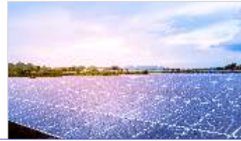
40 MWp Continuum Green Energy Gujarat (Under Commissioning) BATTERY STORAGE EPC PROJECT
