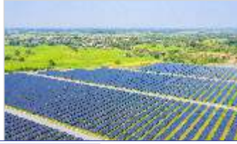
980MWp Greenko Solar Power Project Kumool, Andhra Pradesh (Under Commissioning)
