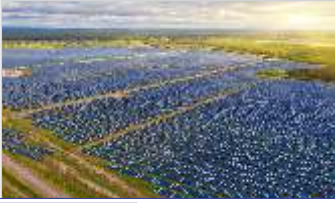
2012MWp Jindal Renewables Bikaner, Rajasthan (Under Commissioning)
