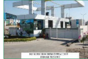
Company : SONIC BIOCHEM EXTRACTION LTD. Capacity : 999 kWp
