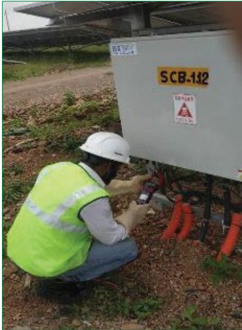
1 MW NTPC, KAWAS, SURAT
