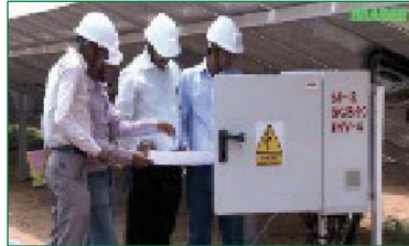
Turnkey EPC Projects Execution
